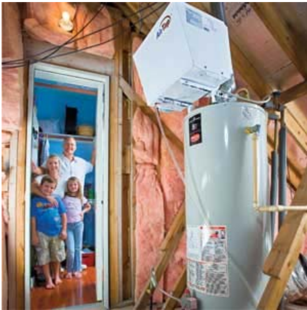
Jim and Rachel King, with kids Jimmy and Ally, retrofitted their water tanks with a heat-pump device and stopped paying for propane.
